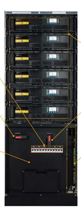
Up to 6 x 50 kW UPS module Integrated UPS module with all UPS essential functions: rectifier, inverter, static bypass, control logic and display.
